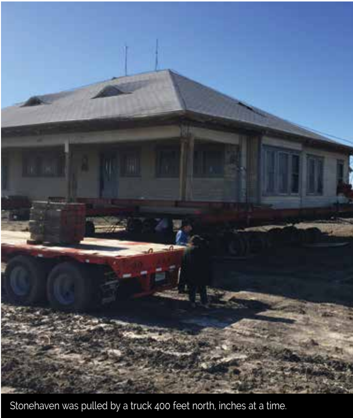
Hydraulic lifts raised the house 18 to 20 inches above its foundation.
