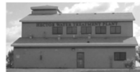
City of Hector Water Treatment Plant
