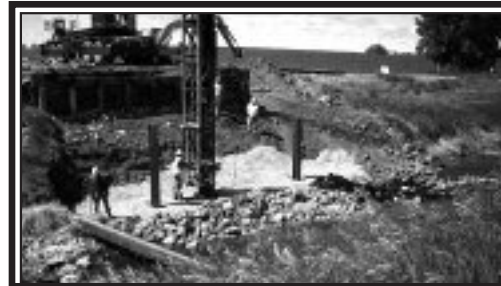
Driving South Pier Line
