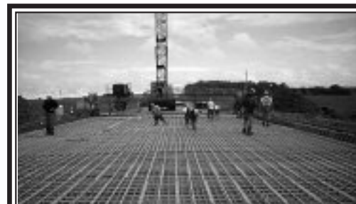
Bridge Deck Work
