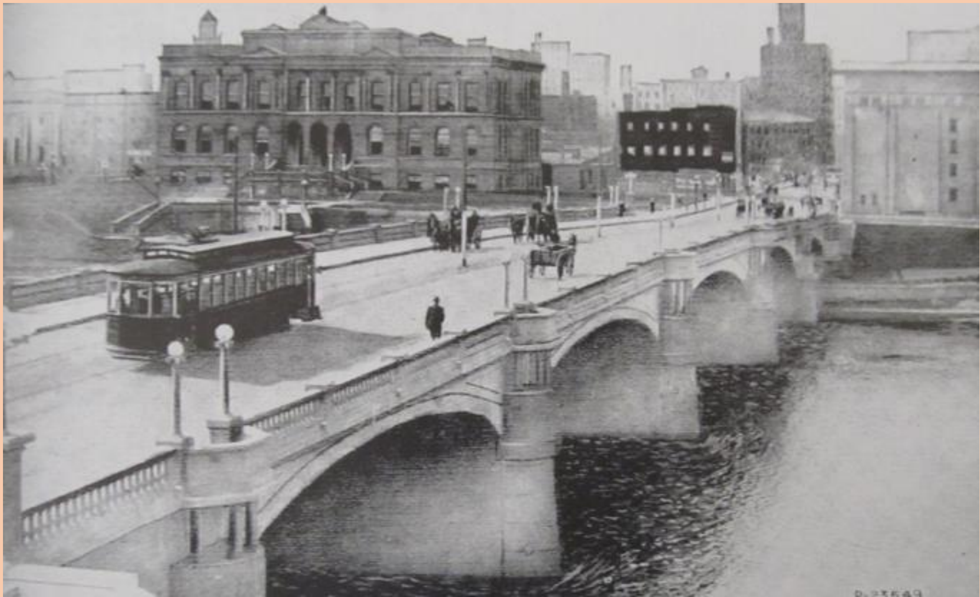
Trolley on Locust Street Bridge. Early trolleys used an electric traction system, with power transferred via overhead wires. This was a safer linkage than the third-rail design used in many subways.
